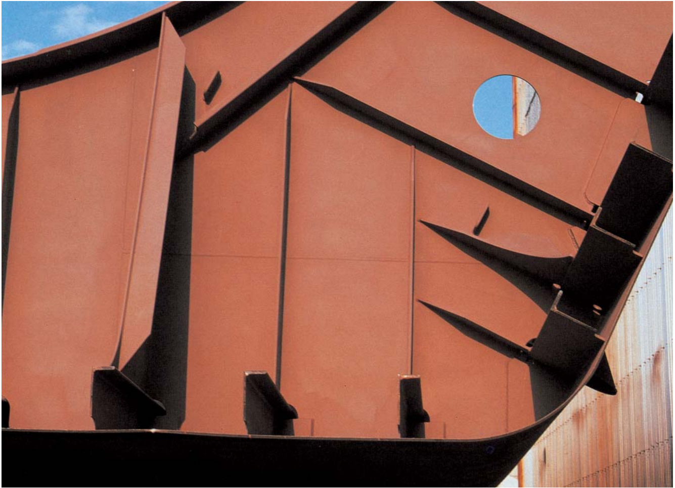
Ships hull block under construction
