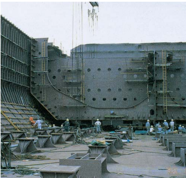
Ship under construction
